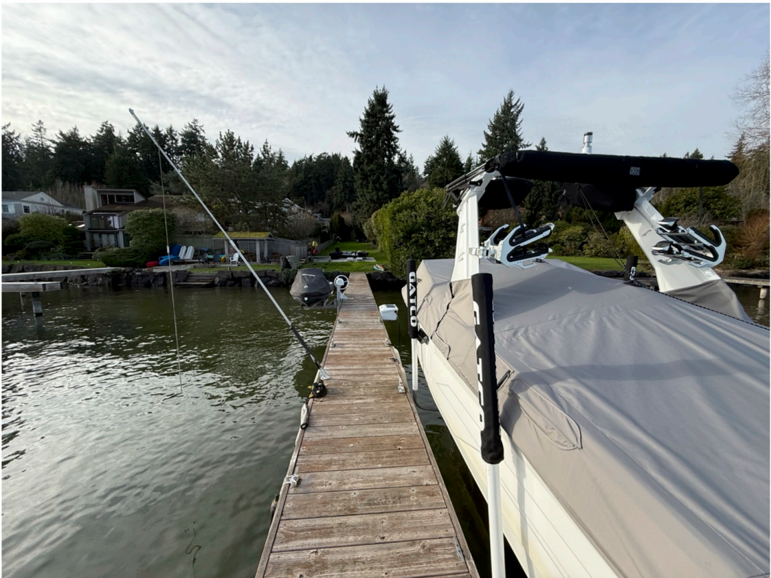
Photo 2 - Existing dock looking landward.
