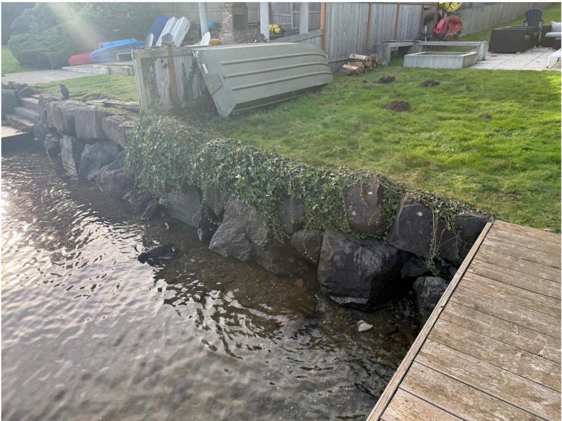
Photo 4 - Existing shoreline south of the dock.
